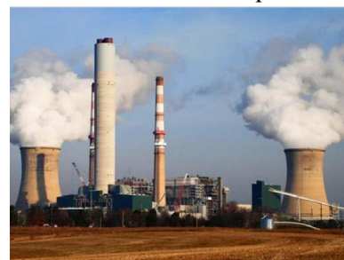
Fig. 1: Self-supporting Rcc Chimney
