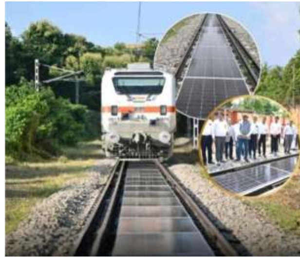
Fig. 1- Solar Panel Installation
