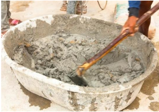
Fig 3.1 Cement mixing
